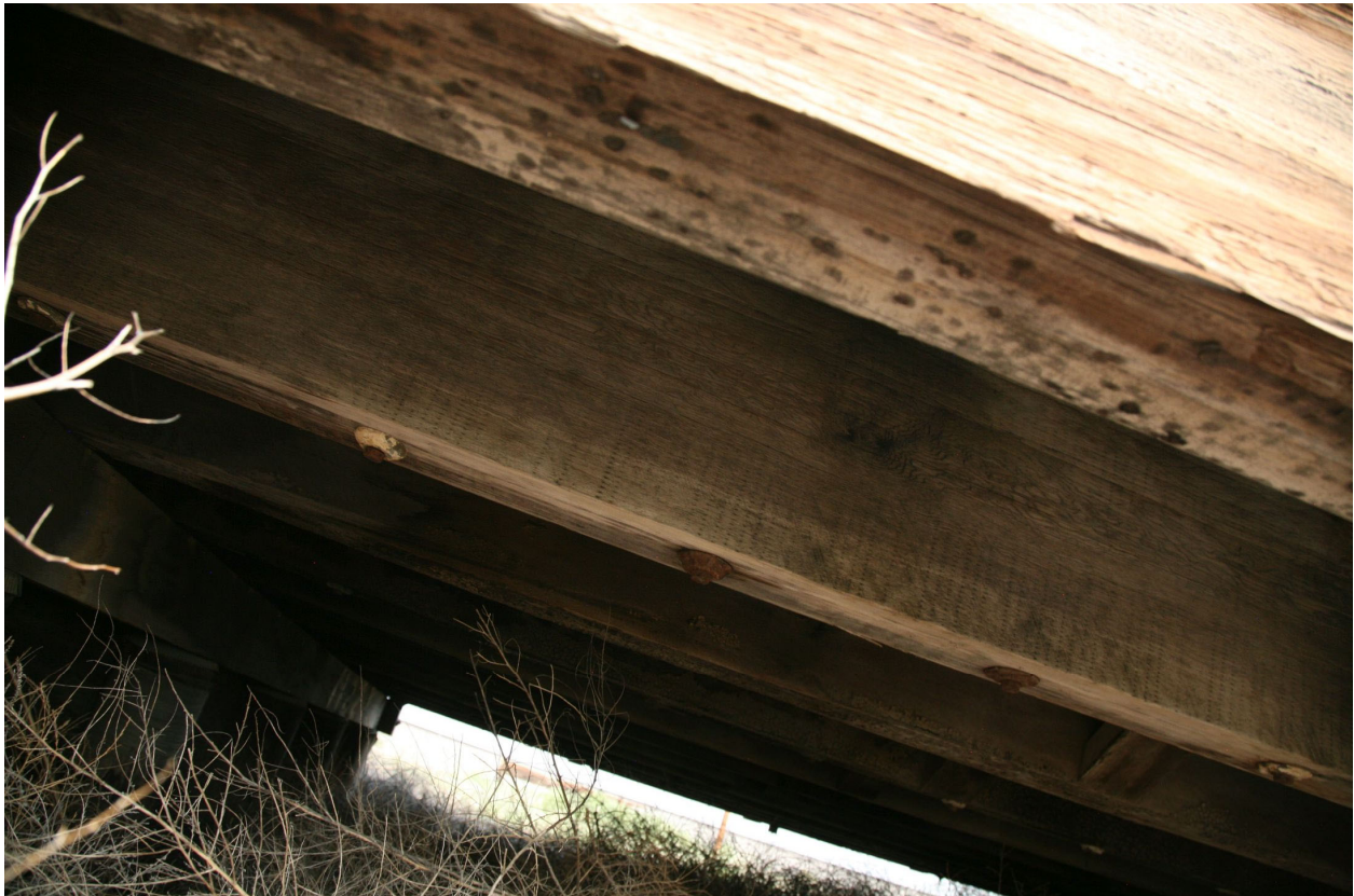
Picture 2 - Repaired Girders
