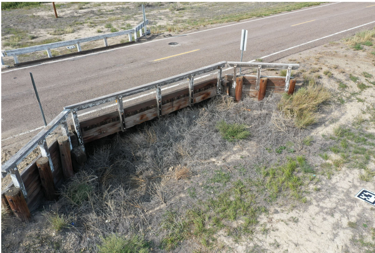
Picture 1 - Bridge M-22-Y
