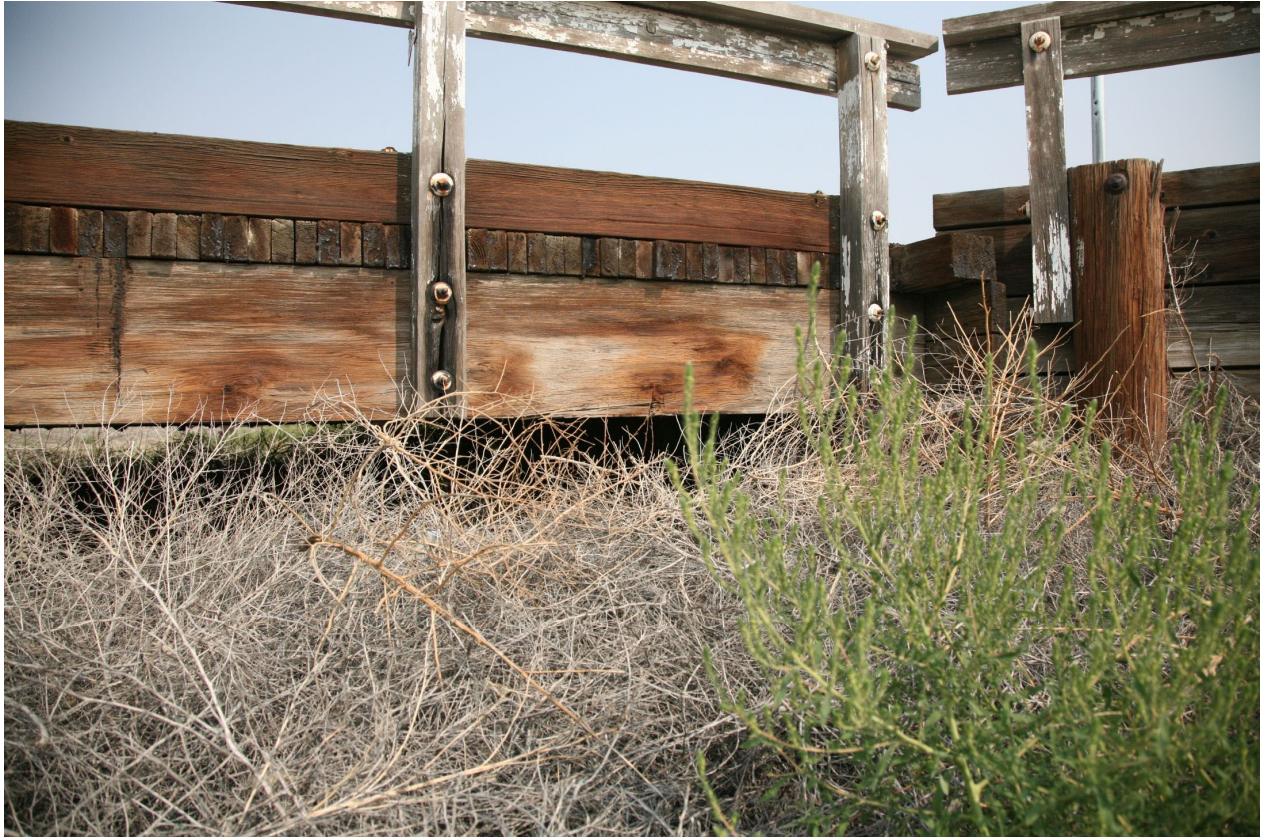
Picture 3 - Girders, Guardrail, Wingwall
